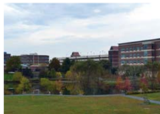
Valley Health Hospital 100+ MOBOTIX Cameras, U.S.A.
