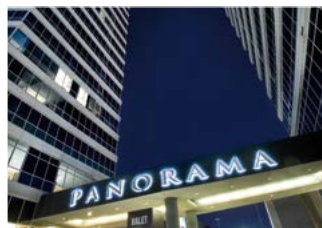
Panorama Towers 137 MOBOTIX Cameras, U.S.A.
