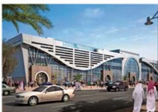
Barwa Commercial Avenue 1,840 MOBOTIX Cameras, Qatar
