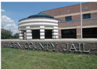
Bergen County Jail 820 MOBOTIX Cameras, U.S.A.
